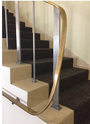
Clockwise from top: Inlaid floor design by Elsa Jemne, wife and partner of Woman's City Club architect Magnus Jemne; Continuous, mobius curve stair railing; Lighting Fixture in the Woman's City Club lecture hall.
